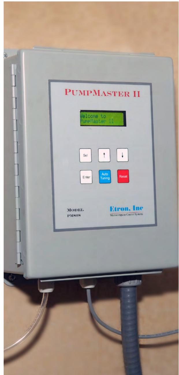
A VARIABLE FREQUENCY DRIVE WAS PLACED ON THE FARM'S MILKING MACHINE VACUUM PUMP, ALLOWING THE VOLUME OF POWER MOVED TO MATCH SYSTEM DEMAND.
